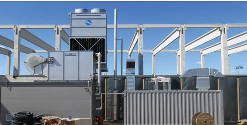
++ In Waren an der Müritz a container style trigeneration plant is constructed. The modular systems can be flexibly expanded and allow more space for production processes
